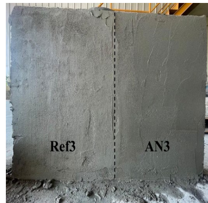
Figure 11. Wall surface plastered with Product C.
