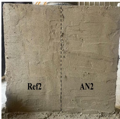
Figure 10. Wall surface plastered with Product B.
